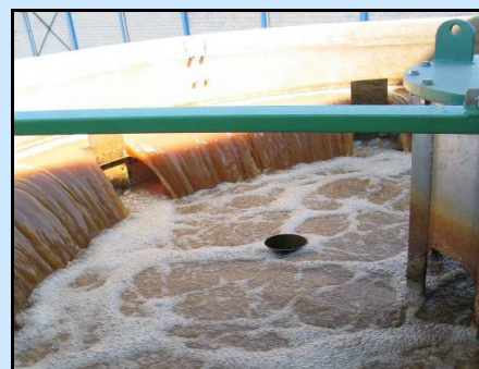
Sanovo Biological Reactor made of fibreglass.
