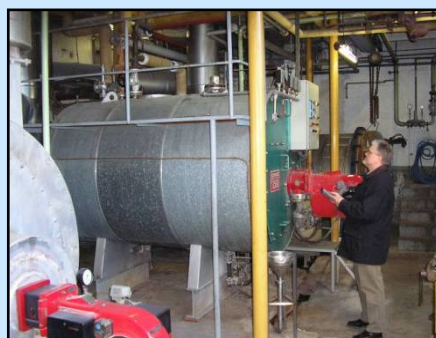
Inspection of boiler for Energy Assessment
