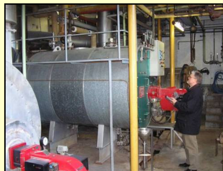
Inspection of boiler for Energy Assessment
